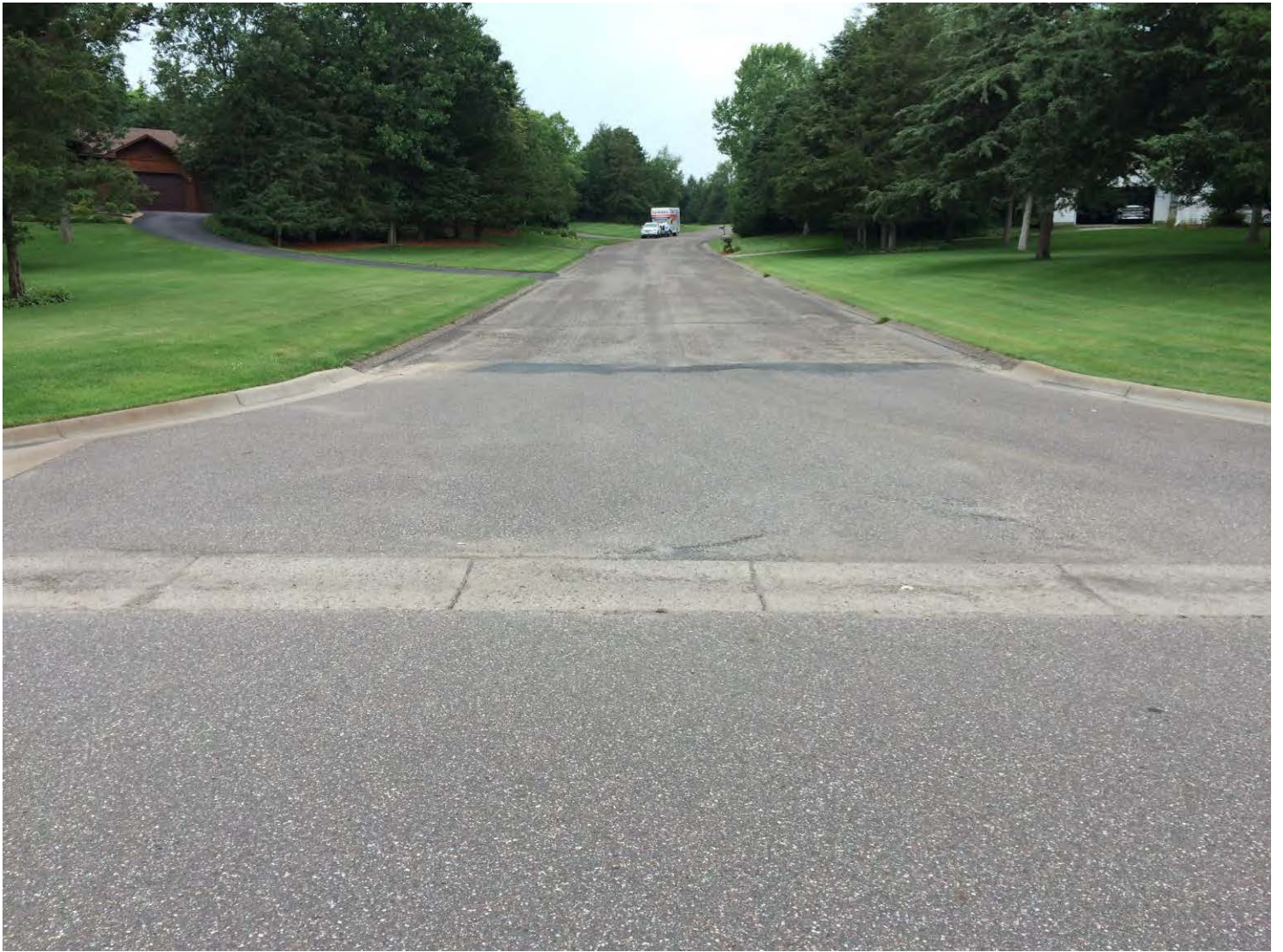
3: 154th Lane from Roanoke Street
