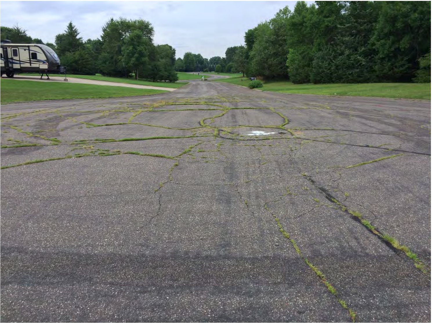
2: Ute Street Cul-de-Sac from the North
