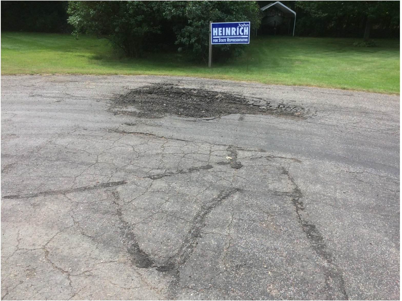
Picture 4: Krypton Street cul-de-sac
