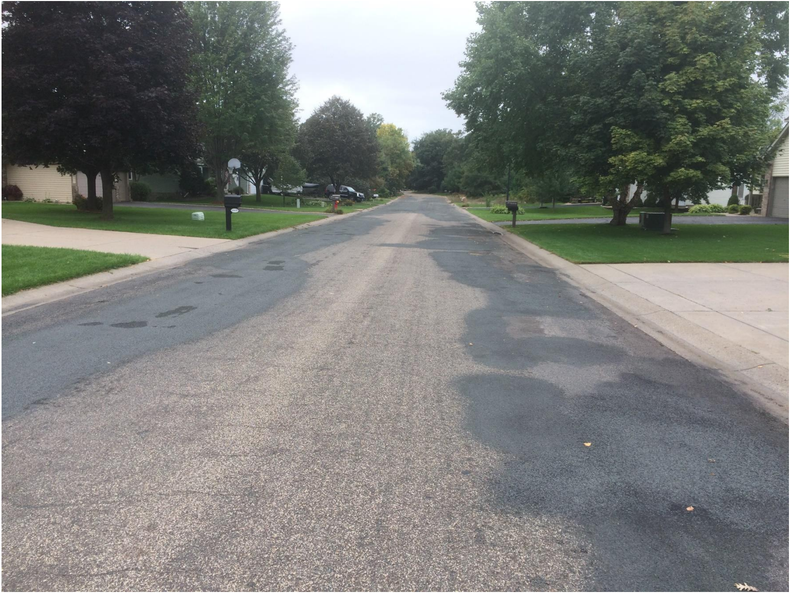
Picture 2: Krypton Street mid-block facing south
