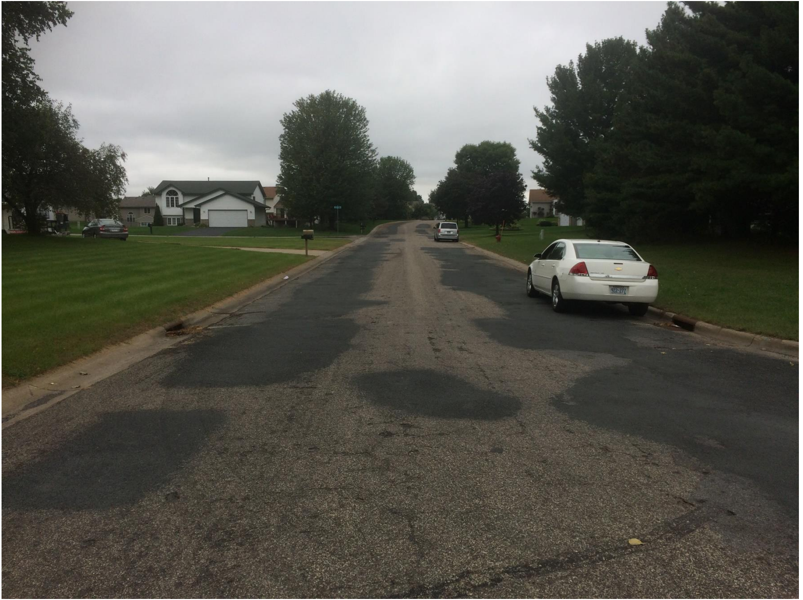
Picture 5: 146 th Avenue from Helium Street, facing west
