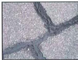
Crack Sealing
