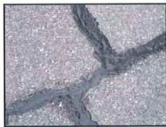
Crack Sealing
