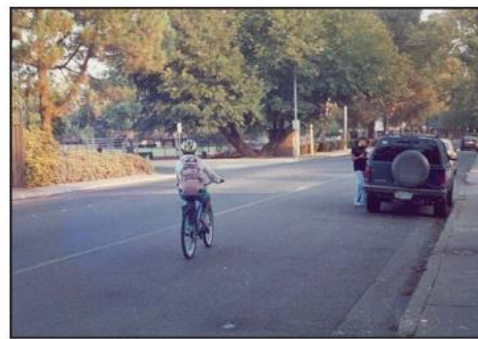
Wide Paved Shoulder Source: www.pedbikeimages.org / Laura Sandt
