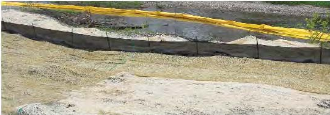
Areas near wetlands, lakes, watercourses or rock outcrops are likely habitat for reptiles and amphibians and may not be suitable for plastic mesh erosion control materials.
