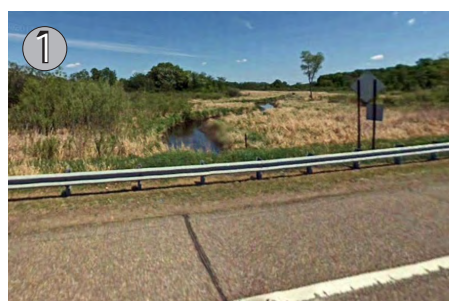
Currently, there is no existing bike trail that connects Armstrong Blvd to Variolite Street. Residents that live in the subdivision that border the Trott Brook do not have access to the scenic creek.
