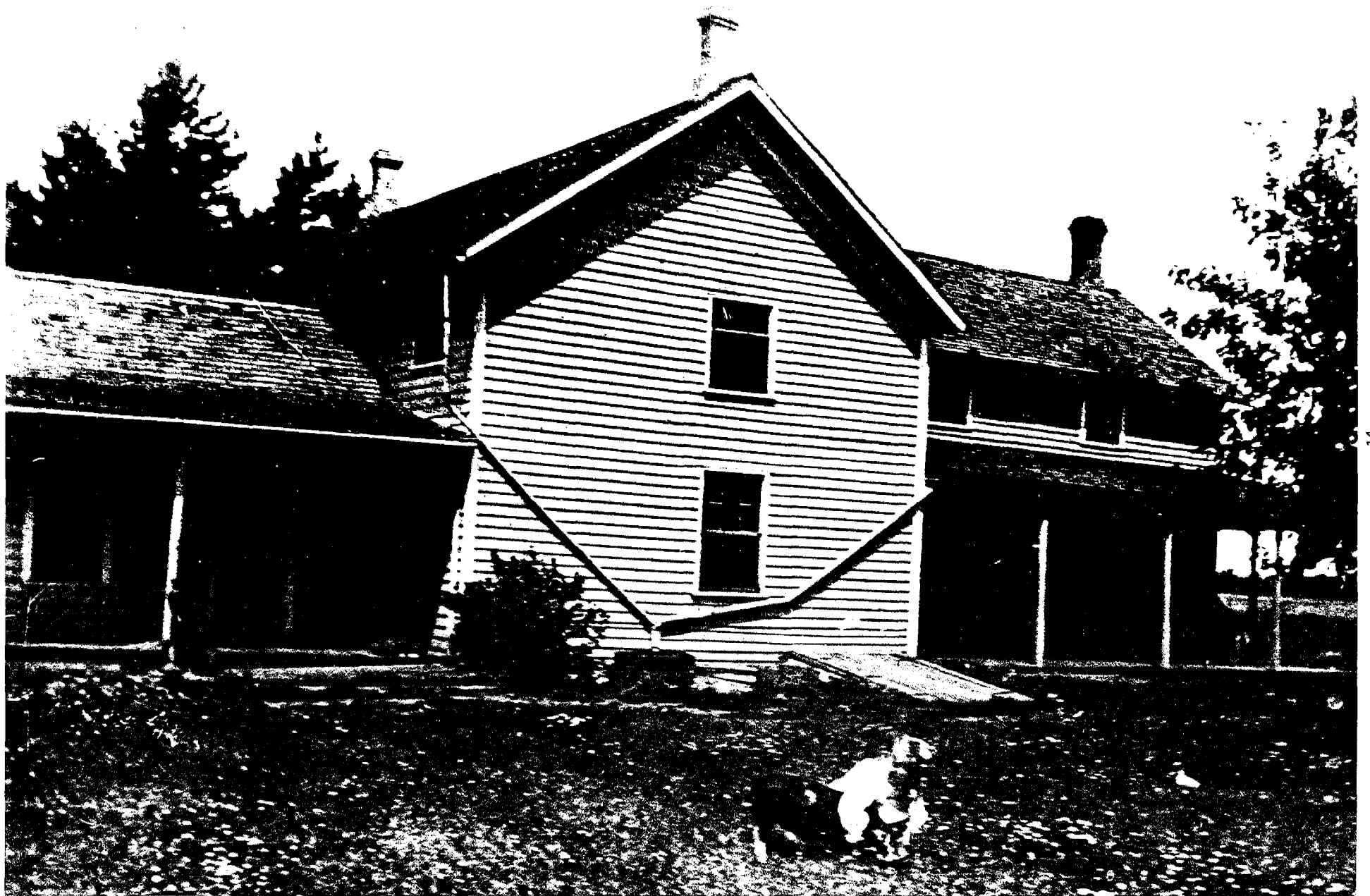
The center part of this building was the original Itasca Hotel.
