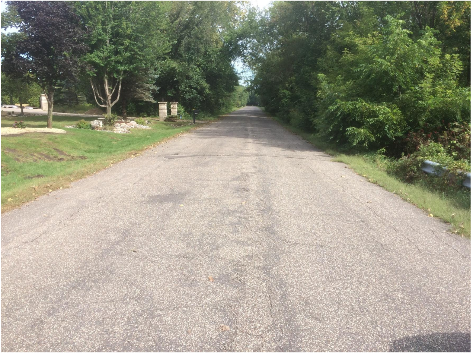
Picture 1: Germanium Street from 170 th Lane
