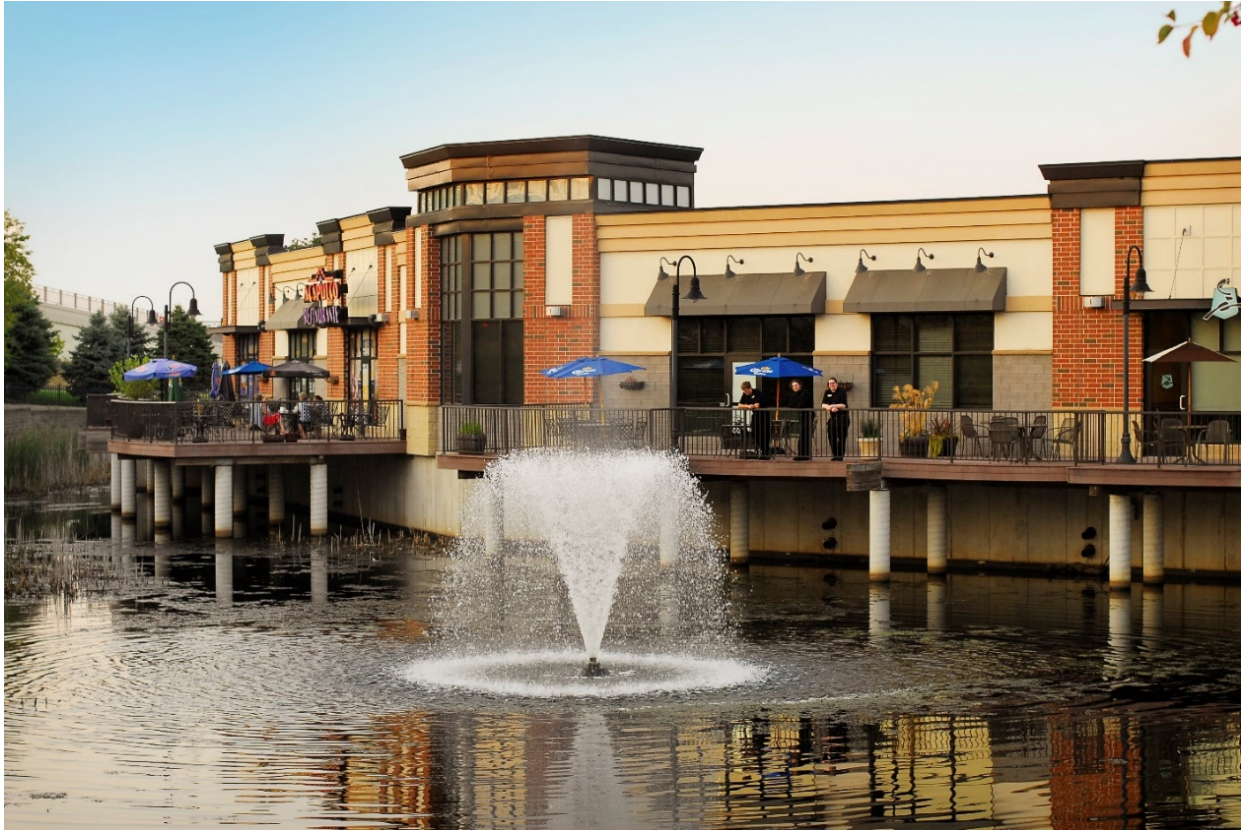
Figure 50: Existing Restaurant Space
