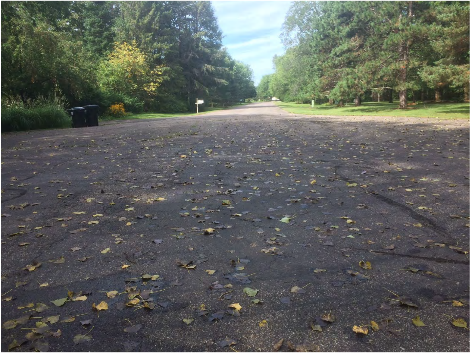
Picture 4: 173 rd Avenue cul-de-sac, looking west
