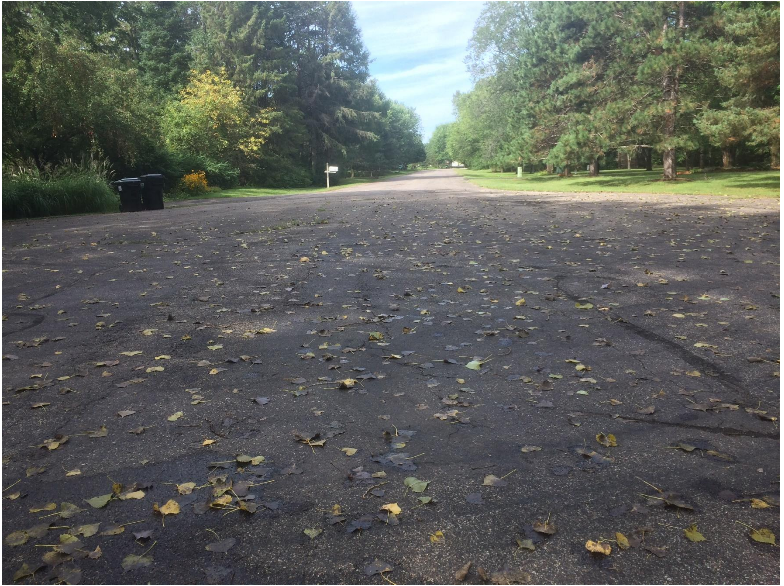
Picture 4: 173 rd Avenue cul-de-sac, looking west
