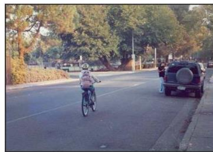
Wide Paved Shoulder Source: www.pedbikeimages.org / Laura Sandt
