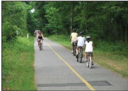
Off-street Facility Source: www.pedbikeimages.org / Laura Sandt
