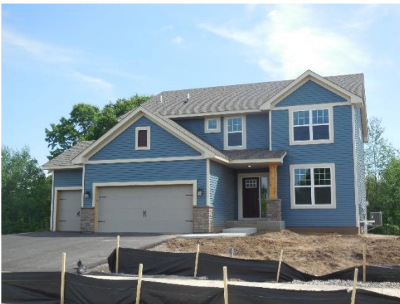
Under Construction Single-Family
