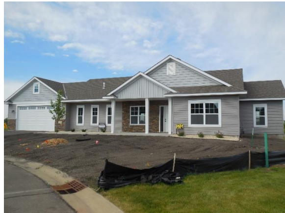
Under Construction Detached Townhome
