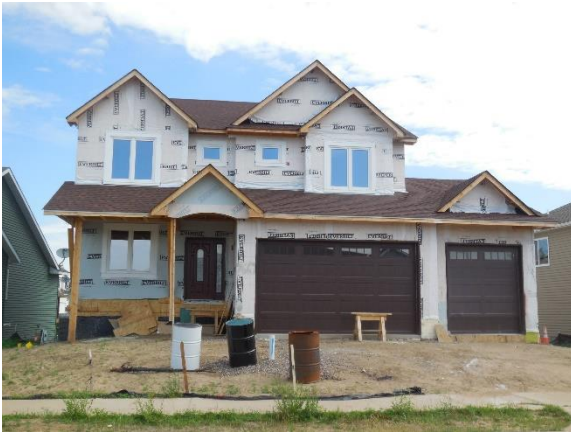
Under Construction Single-Family
