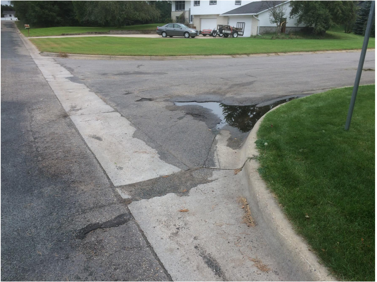
Picture 5: 146 th Avenue valley gutter at Helium Court
