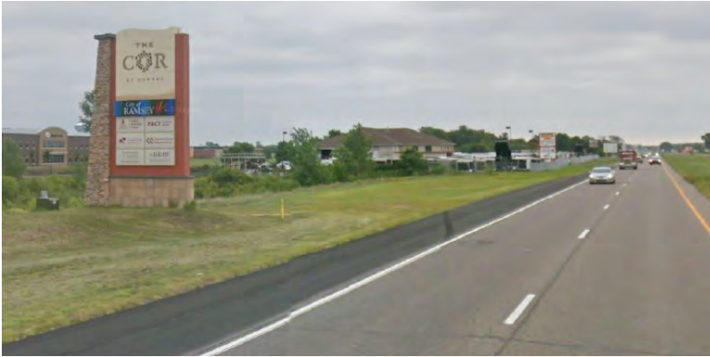
EXISTING X-LARGE SIGNAGE LOCATED ON HWY 10 NEAR CITY HALL
