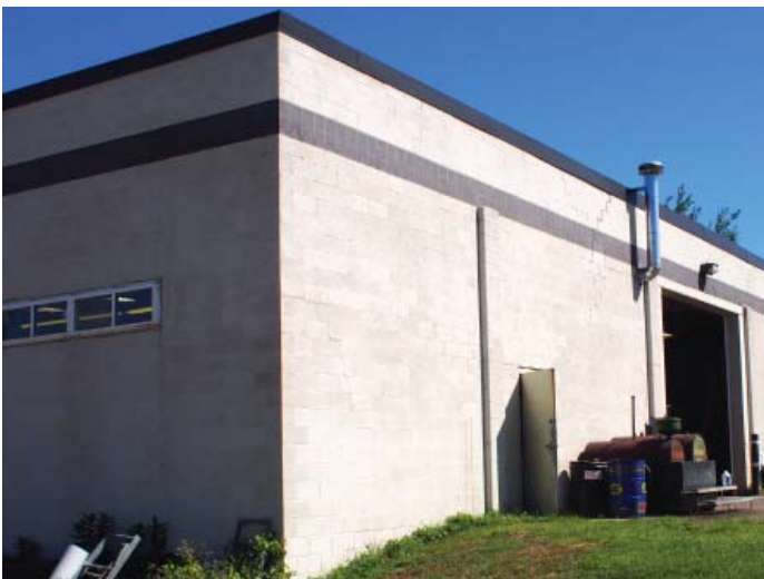
Figure B.3.1: Overall view of Fleet Storage Building
