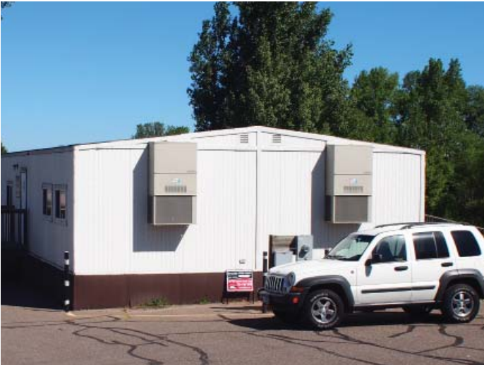
Figure B.5.11: Mechanical systems are in good condition
