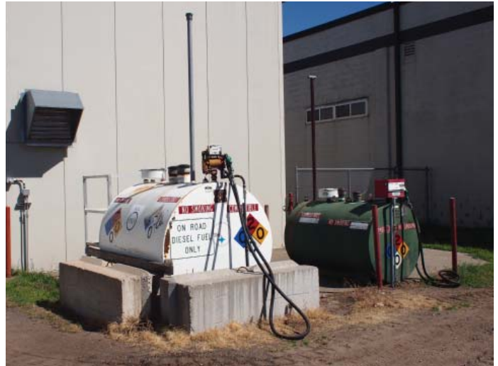
Figure B.7.1: Above ground fuel storage tank
