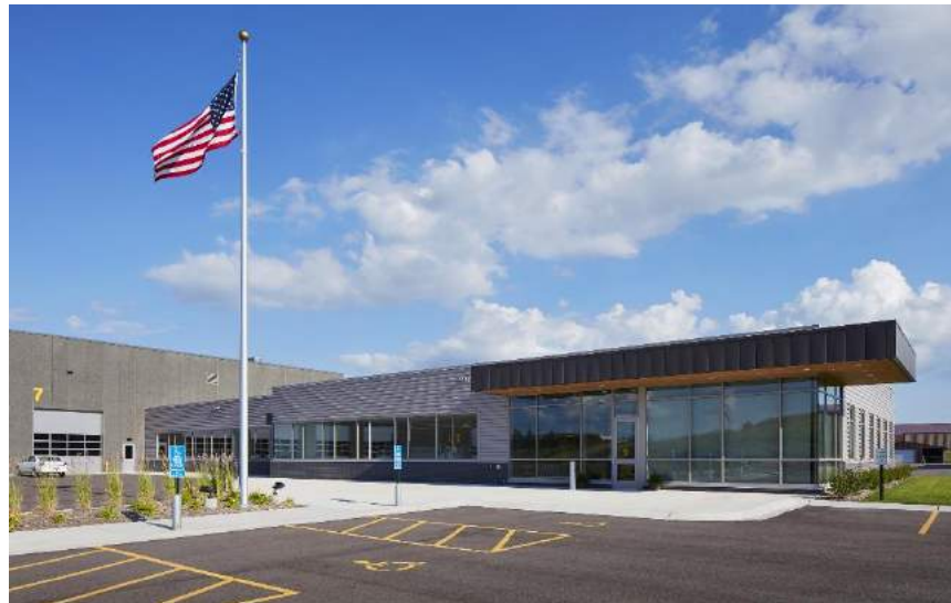
Wright County Highway Department • HCM Architects, 2016
