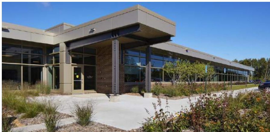
Washington County Public Works – North Shop, Stillwater, MN
