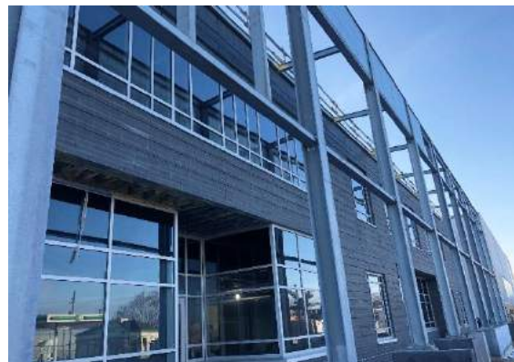
Construction - Two Story Office
