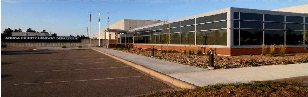
Renovated Office / New Entry
