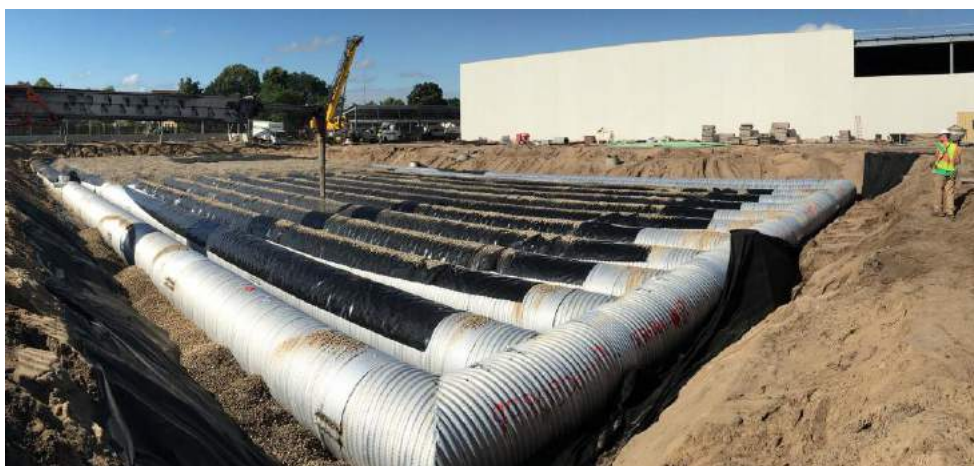
City of Minneapolis East Side Storage & Maintenance Facility – Minneapolis, MN
