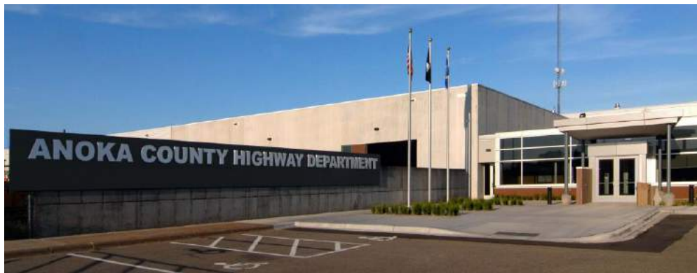
Anoka County Highway Department Facility - Andover, MN
