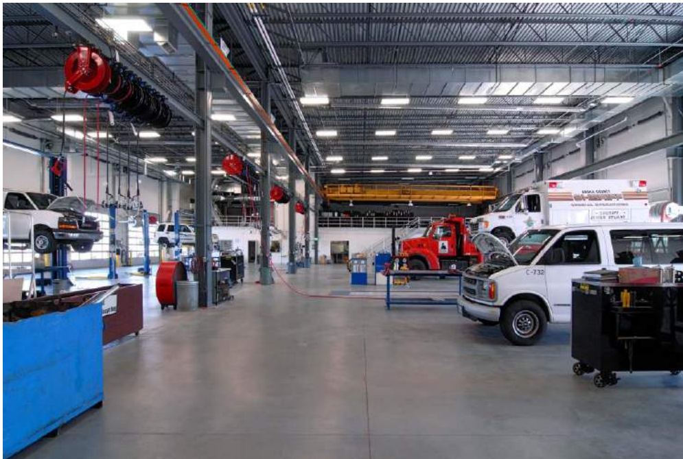
Anoka County Highway Department Facility - Andover, MN
