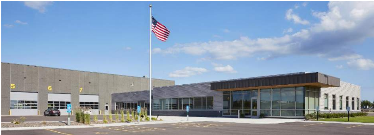
Office / Entry & Fleet Services
