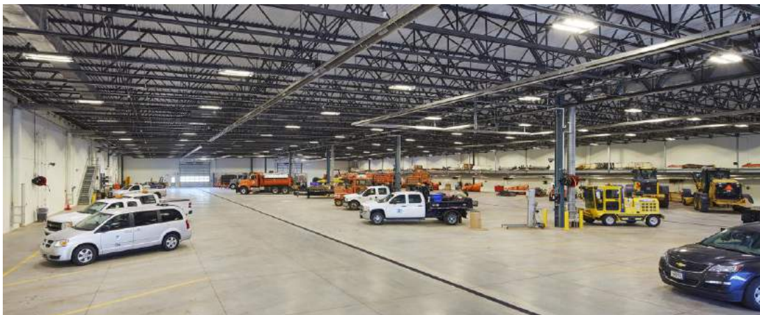
Wright County Highway Department - Vehicle Warm Storage
