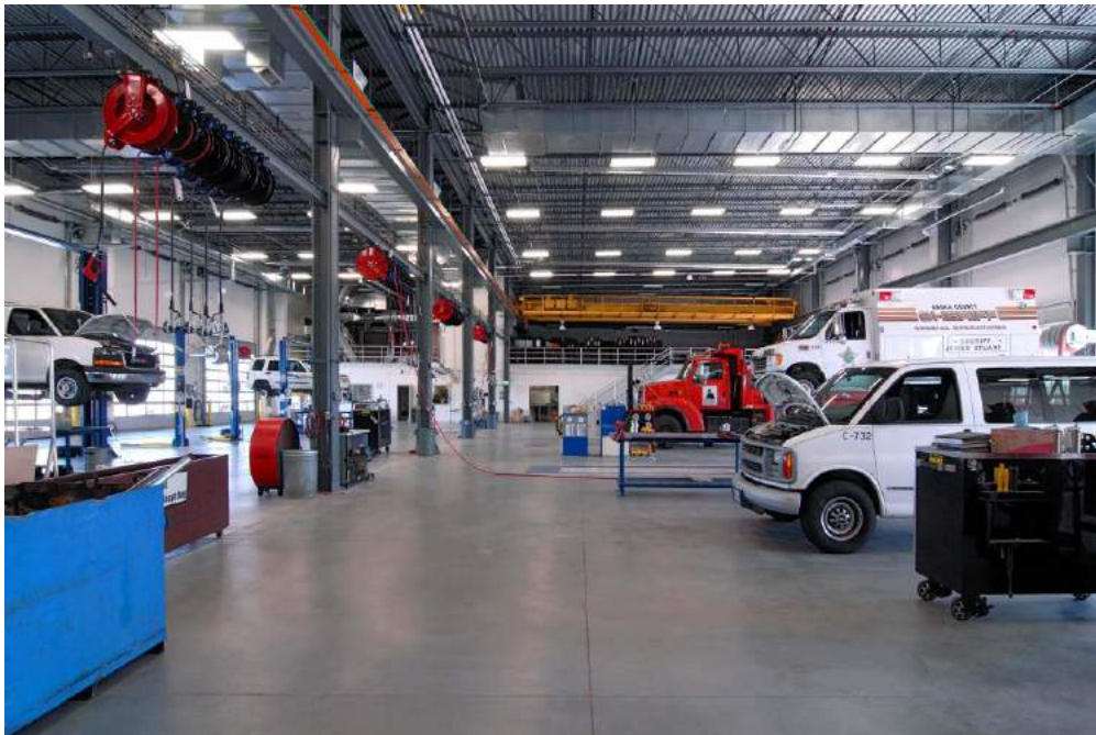
Anoka County Highway Department Facility - Andover, MN
