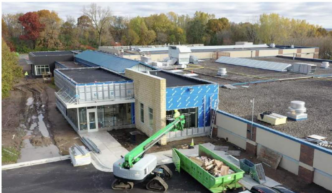
City of Woodbury Public Works - Woodbury, MN
