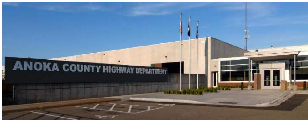
Anoka County Highway Department Facility - Andover, MN
