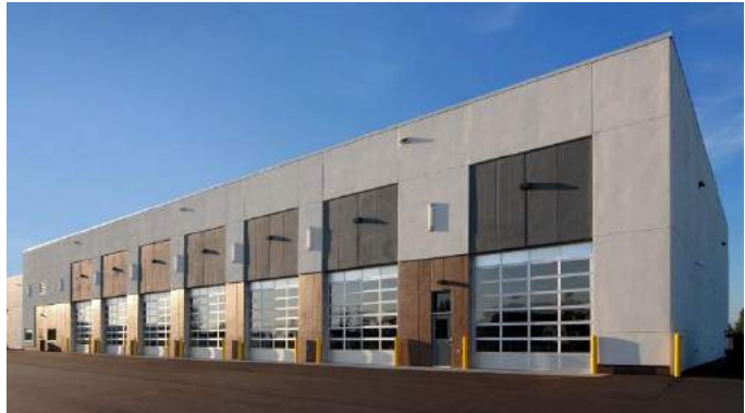
New Fleet Services Addition
