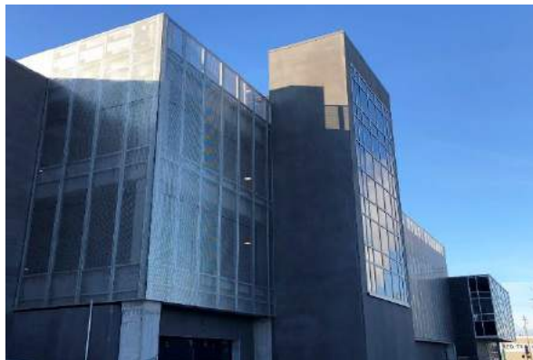
Construction - Parking Ramp
