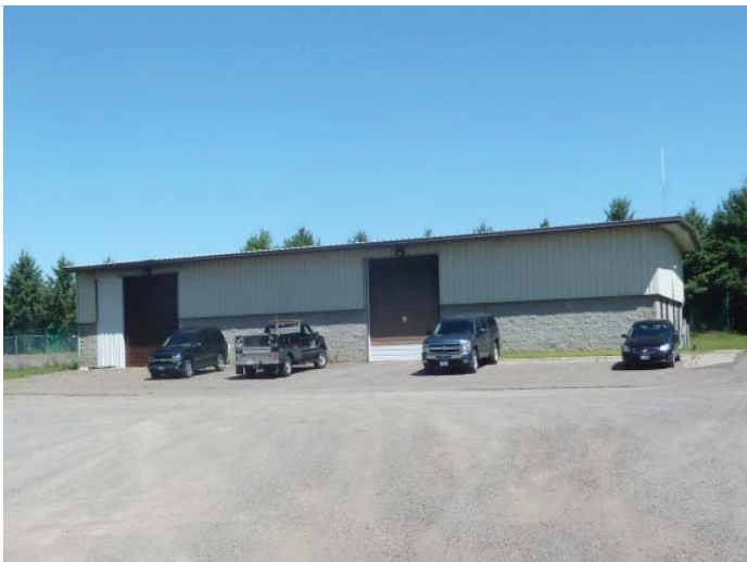
Figure B.1.1: Overall view of Utility and Sign Shop Building
