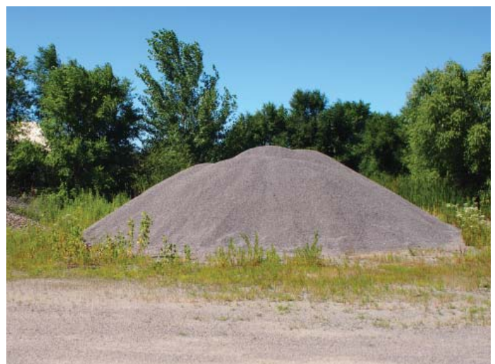
Figure B.6.5: Granular storage areas do not meet current EPA standards for cover
