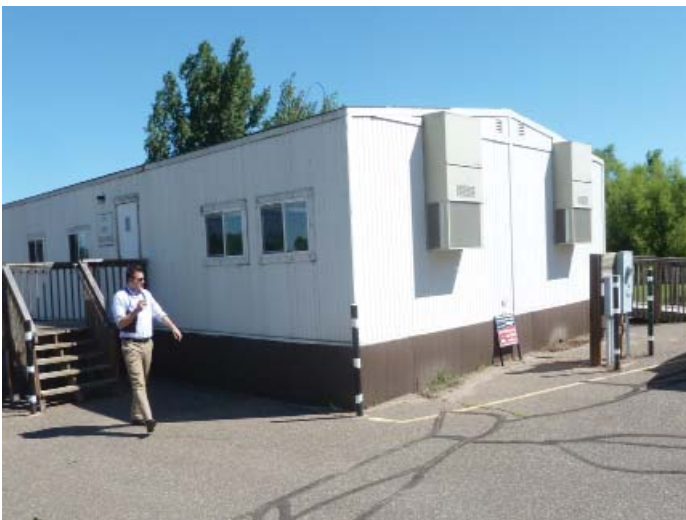
Figure B.5.1: Overall view of Administration Trailer
