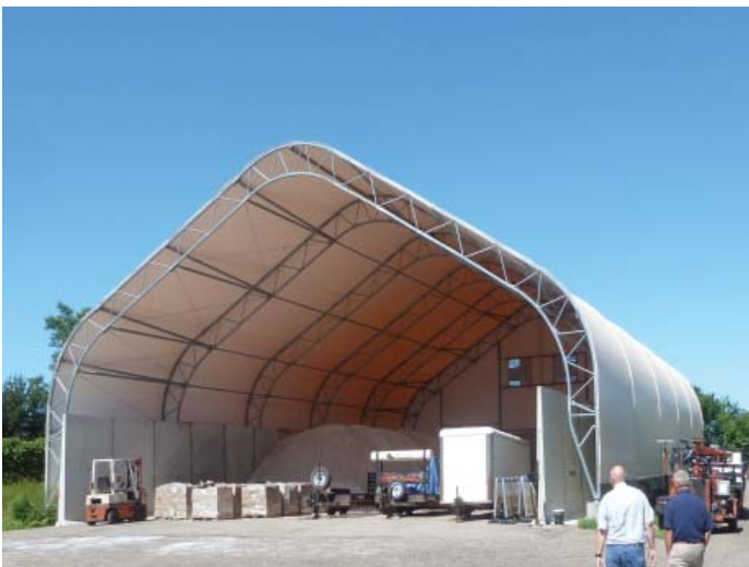
Figure B.4.1: Overall view of Salt Storage Building
