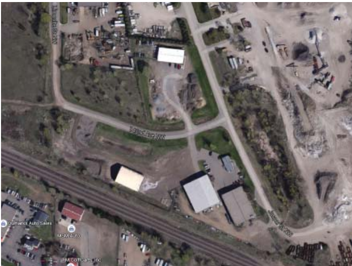
Figure B.6.1: Aerial view of Public Works site
