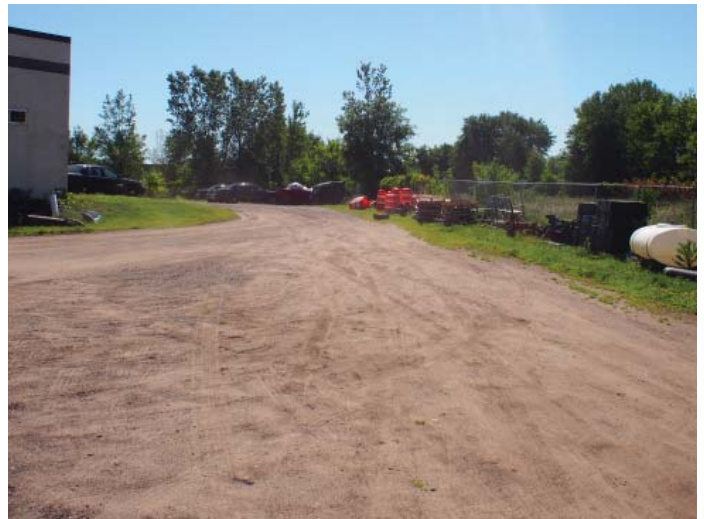
Figure B.6.4: Unpaved areas of site are in good condition with no signs of deep rutting
