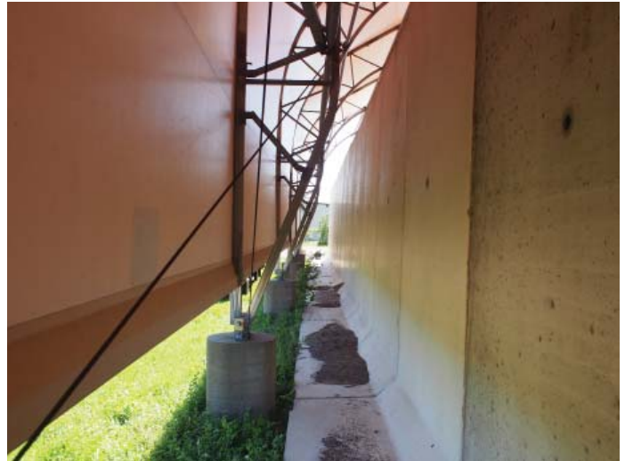
Figure B.4.2: Precast wall panels and concrete foundation piers along exterior wall are in good condition
