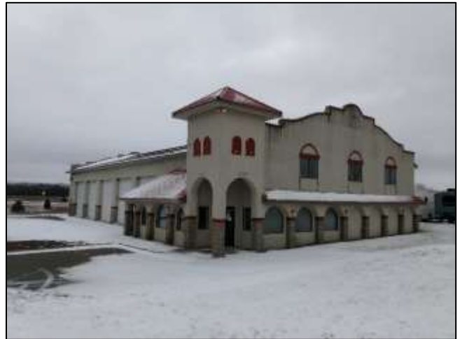
Looking south on Interstate 94
