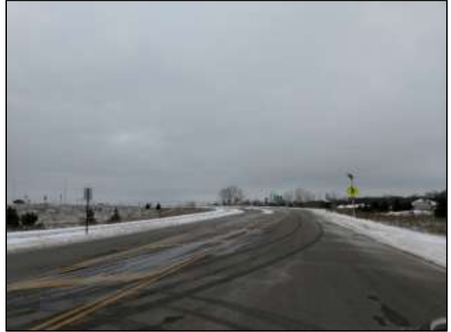
Looking east on Riverdale Drive Northwest
