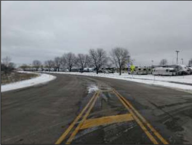
Looking west on Riverdale Drive Northwest
