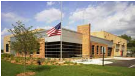
ST. ANTHONY PUBLIC WORKS FACILITY St. Anthony, MN
