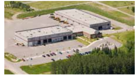
ELY JOINT USE MAINTENANCE FACILITY Ely, MN
