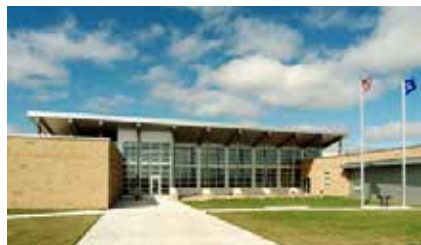
CITY OF BEMIDJI PUBLIC WORKS FACILITY Bemidji, MN
