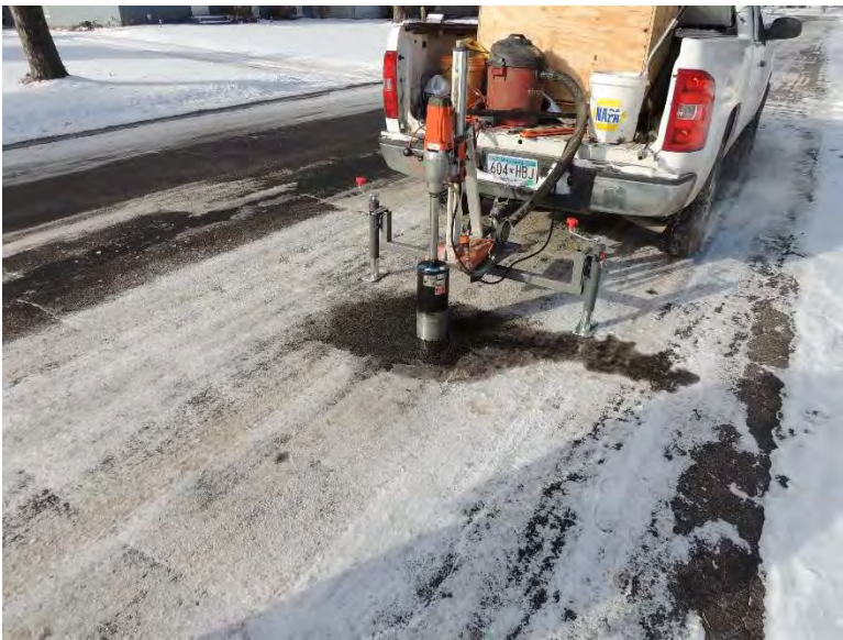
Figure I-10. Coring operations and sample core extracted from Ingberg Trail in Cottage Grove, MN
