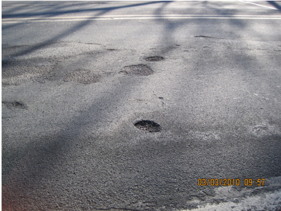
Figure 1: Stripping of asphalt pavement under chip seal.
