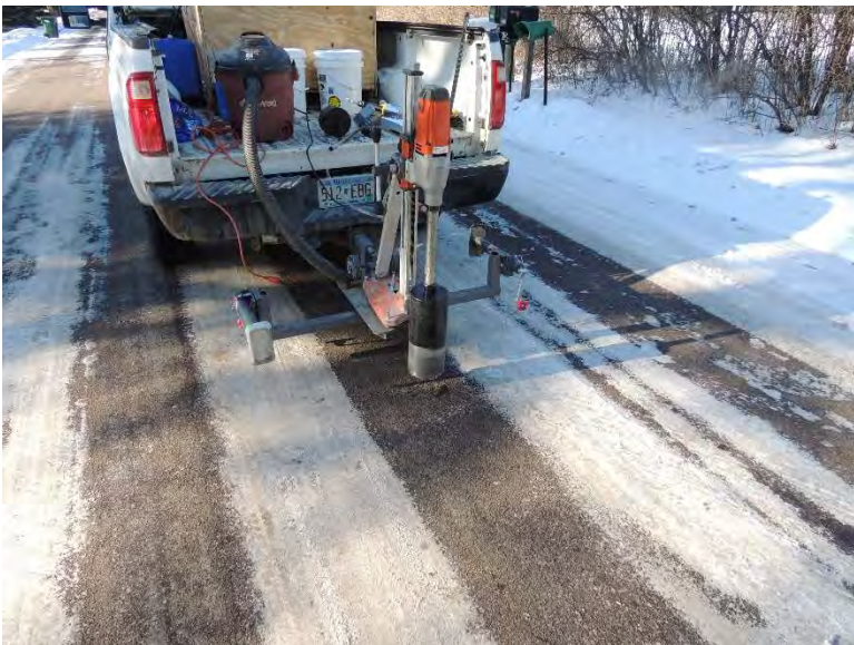
Figure I-2. Coring operations and sample core extracted from the east end of 93rd Avenue in Blaine, MN
