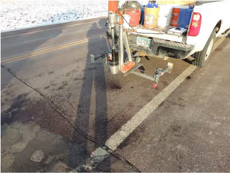
Figure I-15. Coring operations and sample core extracted from the south part of CSAH 9 in Sibley County, MN
