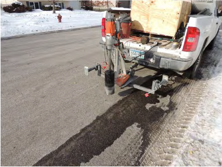
Figure I-11. Coring operations and sample core extracted from Jensen Ave in Cottage Grove, MN
