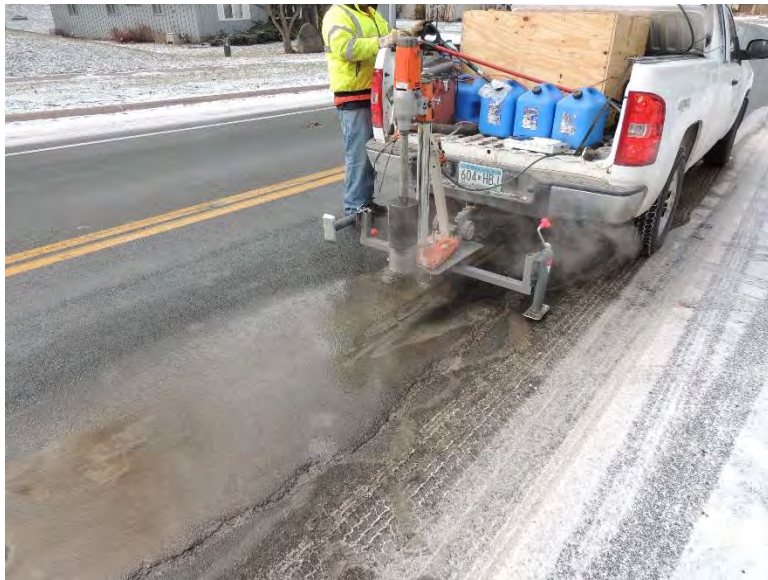
Figure I-6. Coring operations and sample core extracted from 134th Street in Burnsville, MN
