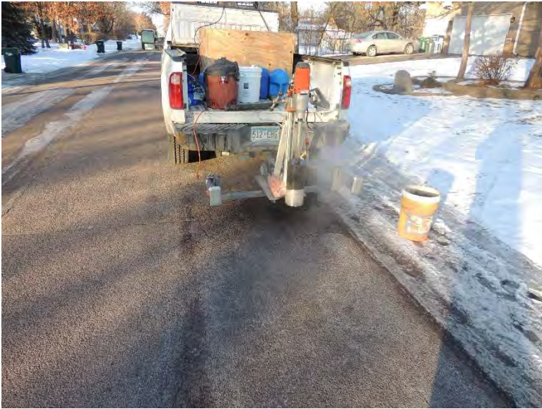
Figure I-1. Coring operations and sample core extracted from the east end of 93rd Avenue in Blaine, MN
