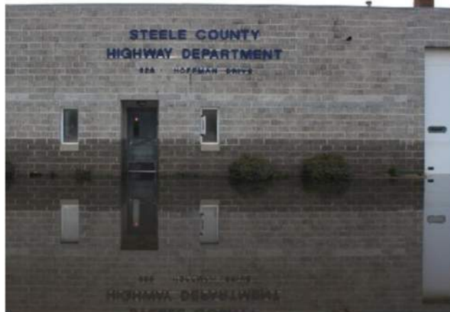
Below: A view of the existing flooded facility
