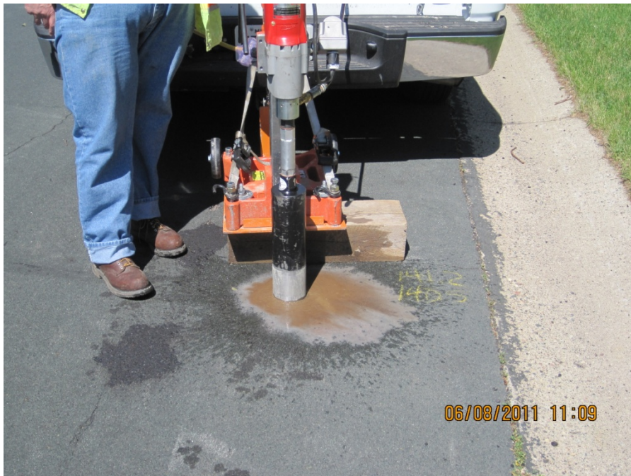
Figure 15 Coring at NI location
