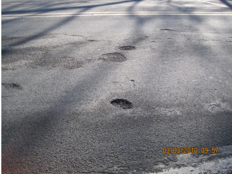
Figure 1: Stripping of asphalt pavement under chip seal.
