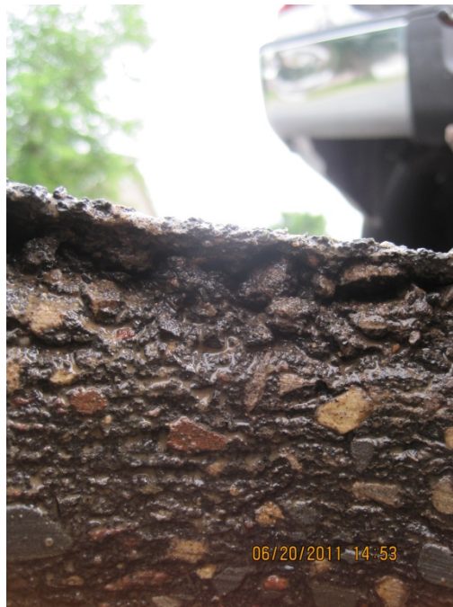
Figure 18 Pavement in area of stripping
