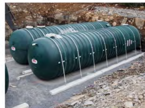
Exhibit 3: Example underground fiberglass storage tanks (Xerxes).
