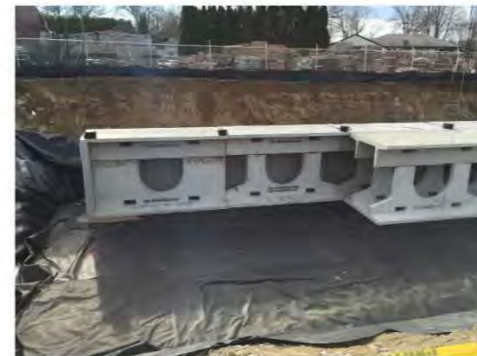
Exhibit 2: Example concrete vault storage tank (StormTrap).
