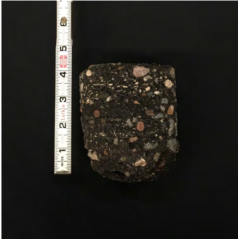
SB-37 Core Photograph
