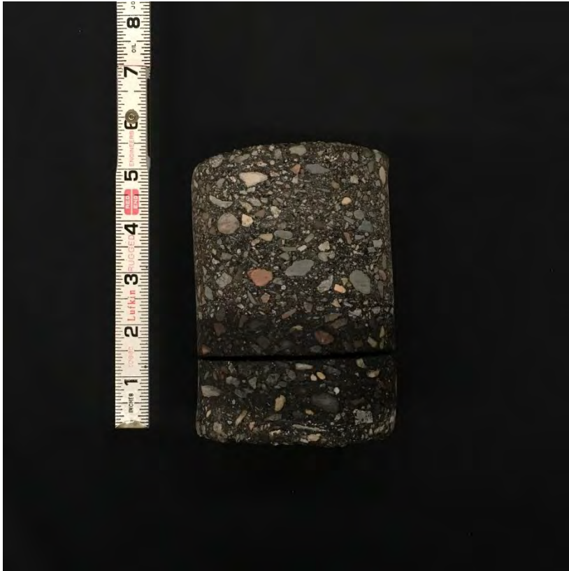
SB-47 Core Photograph
