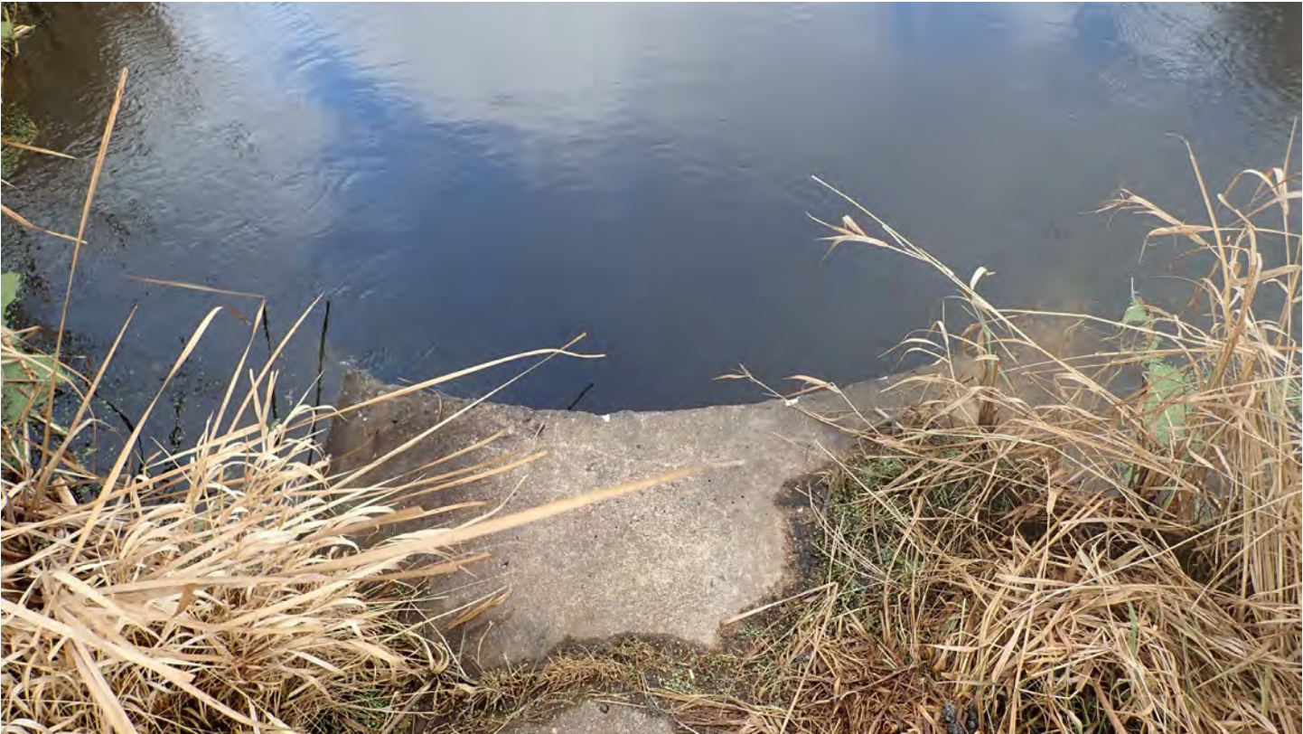
P8: Trott Brook Culvert End
