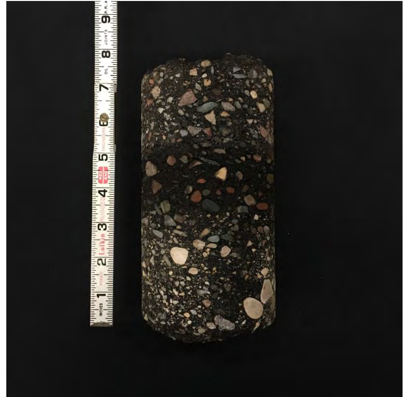
SB-26 Core Photograph
