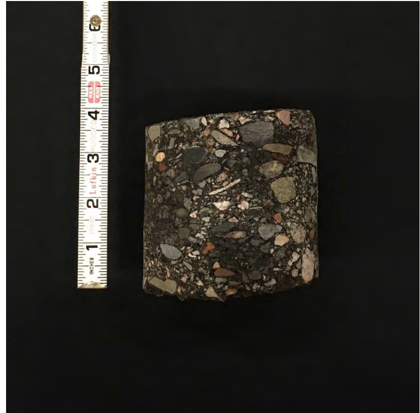
SB-30 Core Photograph
