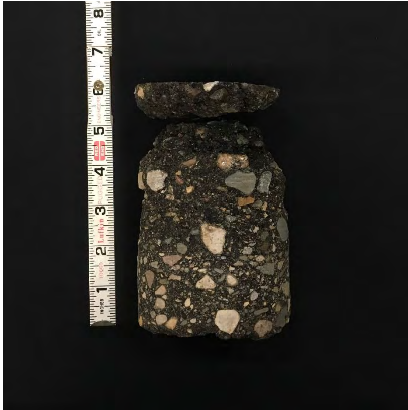
SB-9 Core Photograph
