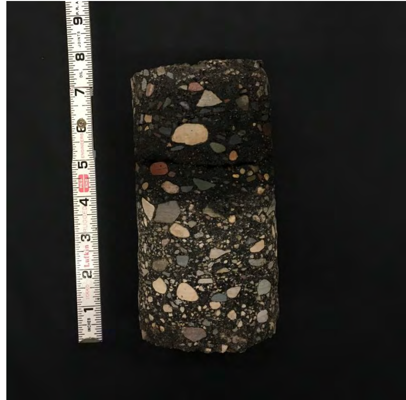
SB-48 Core Photograph
