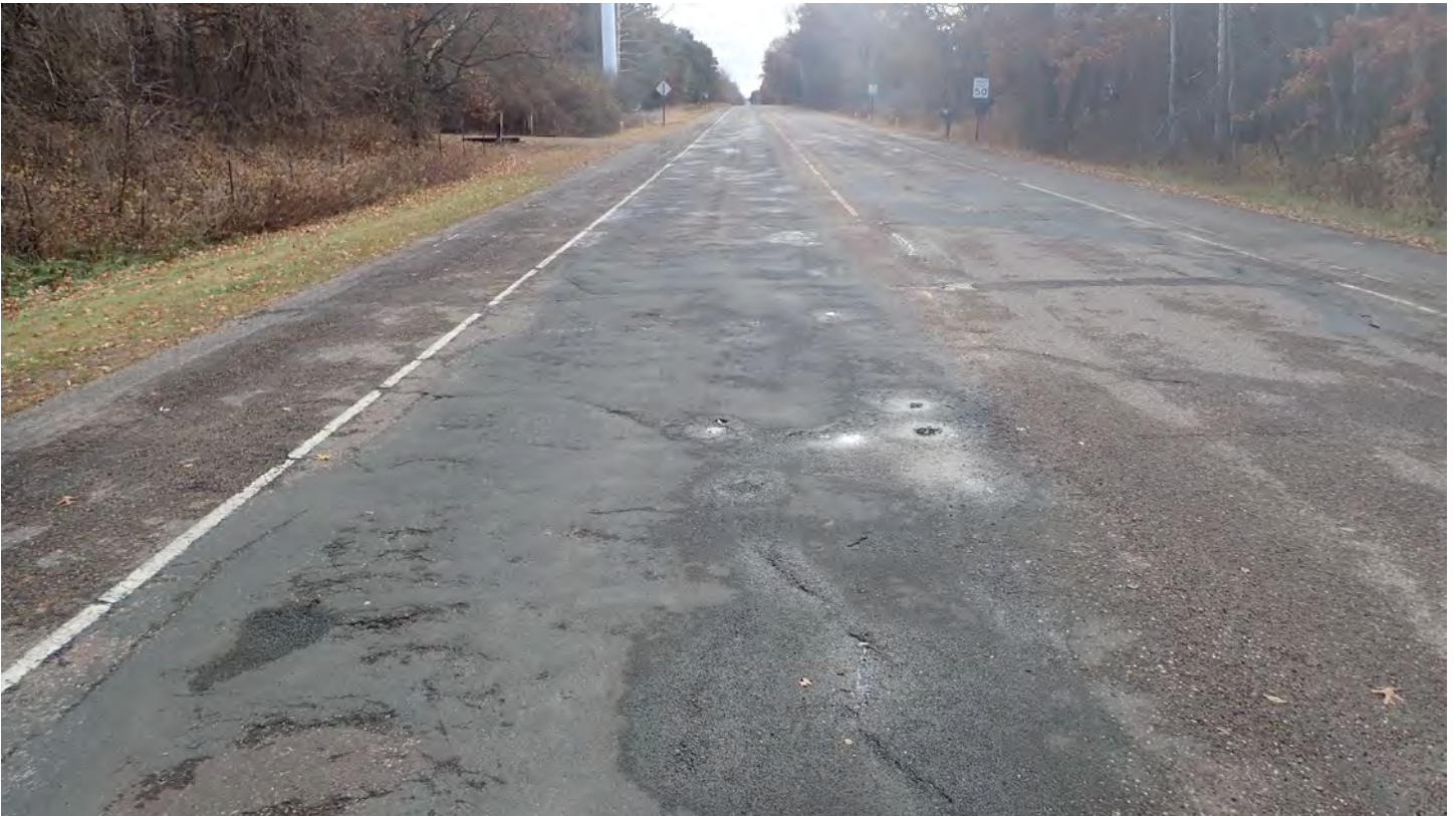
P11: Variolite south of 173 rd Ave – facing south
