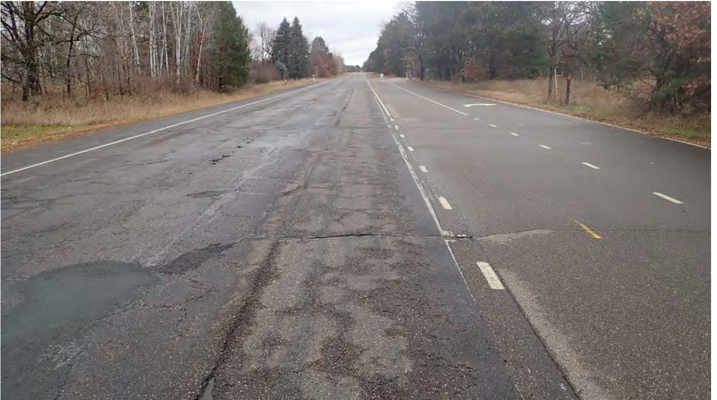
P2: Variolite south of 159 th Ave – facing north
