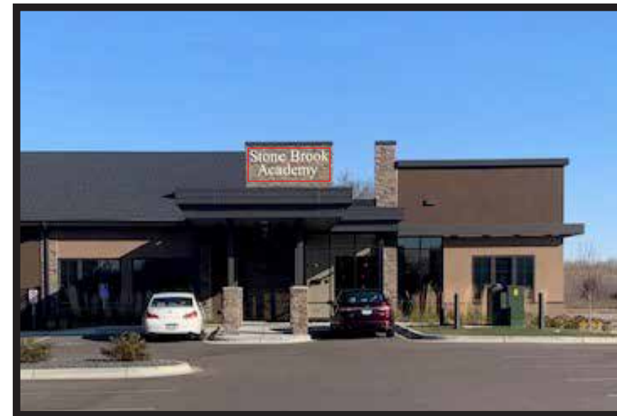
Existing Sign to be Removed
