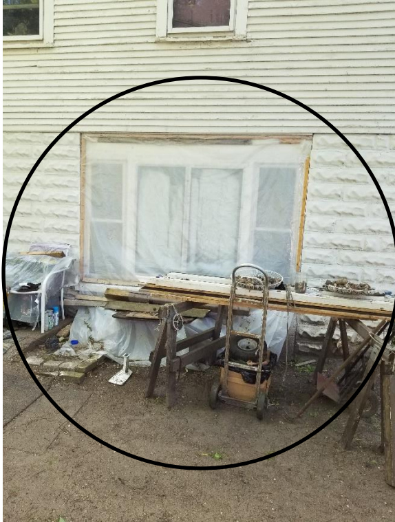
Exhibit 5: Work being done on window on south side of home
