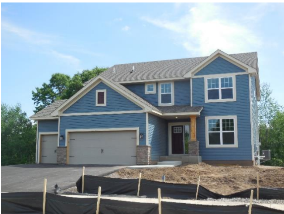
Under Construction Single-Family
