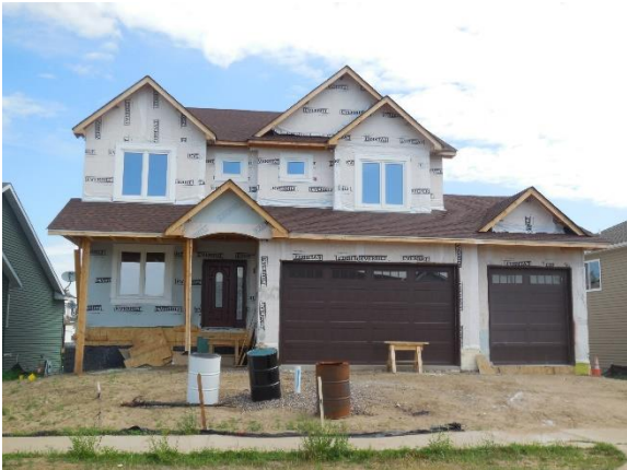
Under Construction Single-Family
