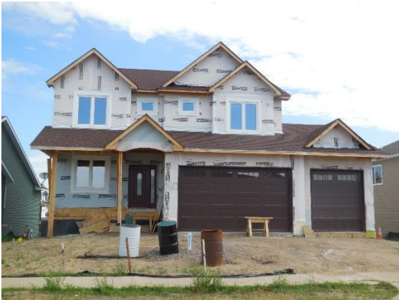
Under Construction Single-Family
