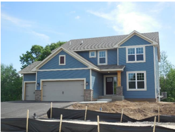
Under Construction Single-Family
