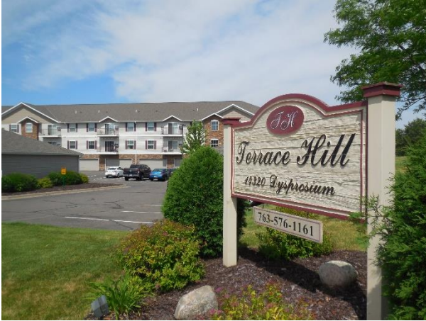
Terrace Hill Apartment 14320 Dysprosium Street NW
