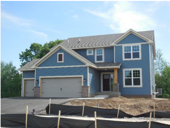
Under Construction Single-Family
