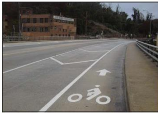
Buffered Bicycle Lane Source: www.pedbikemages.org / Lyubov Zuyeva
