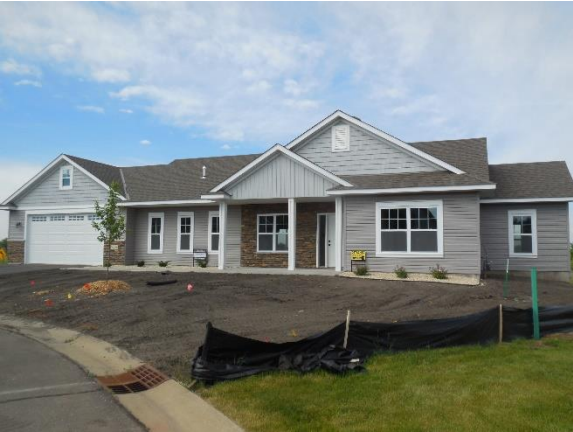
Under Construction Detached Townhome
