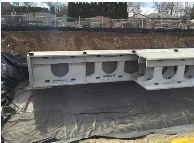
Exhibit 2: Example concrete vault storage tank (Storm Trap).
