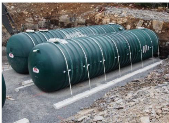
Exhibit 3: Example underground fiberglass storage tanks (Xerxes).
