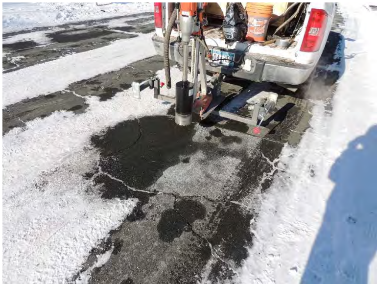
Figure I-18. Coring operations and sample core extracted from Newbury Alcove straight portion in Woodbury, MN
