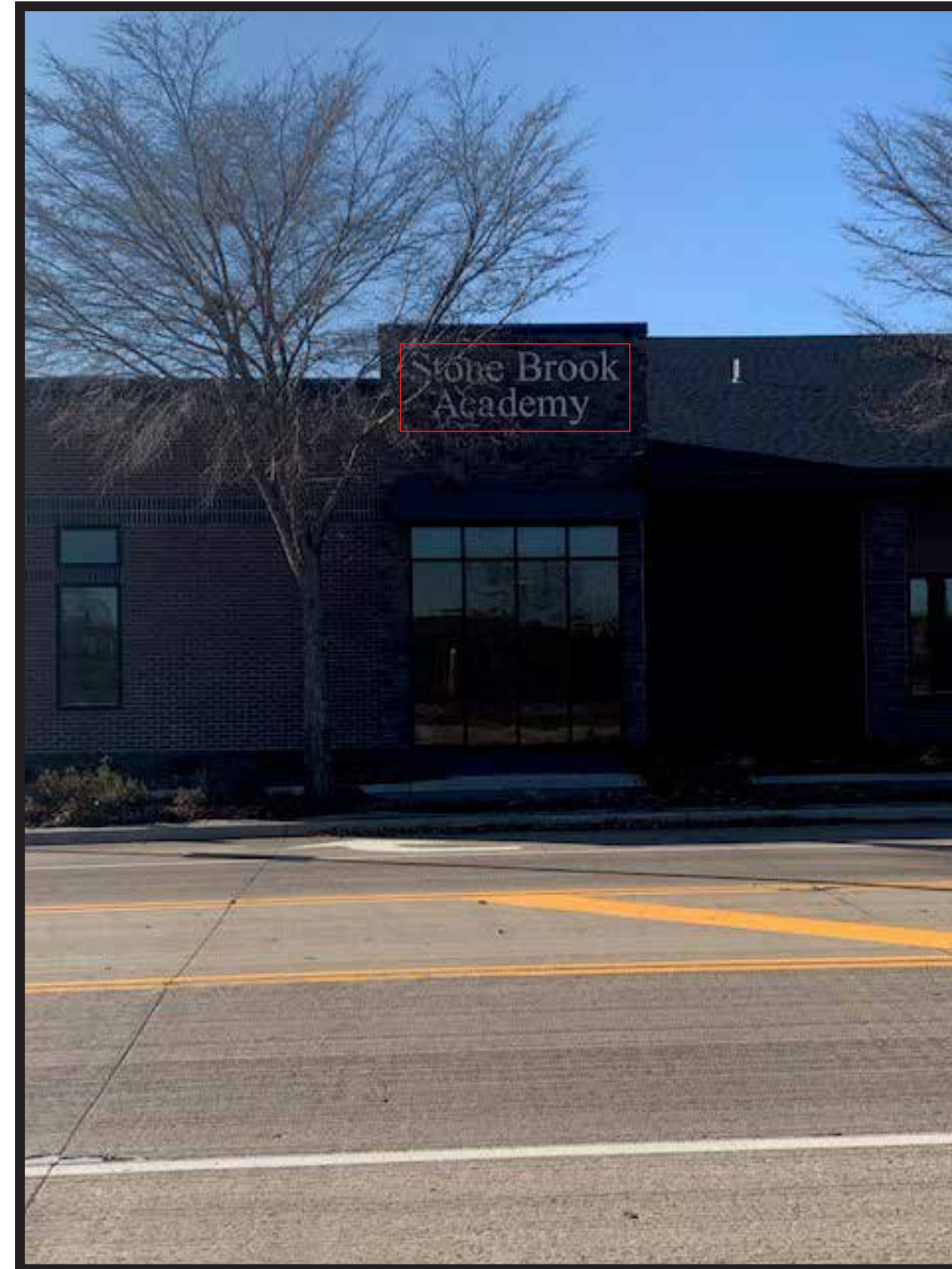
Existing Sign to be Removed
