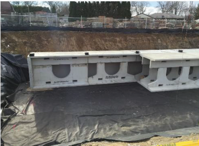
Exhibit 2: Example concrete vault storage tank (Storm Trap).
