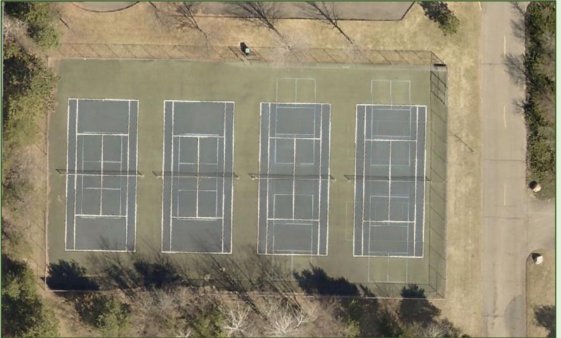
Existing Courts at Loral I Armstrong Delaney Central Park
