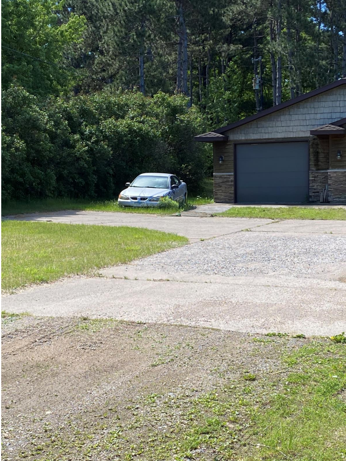
Exhibit 1-2: Evidence of Violation (5.28.21)
