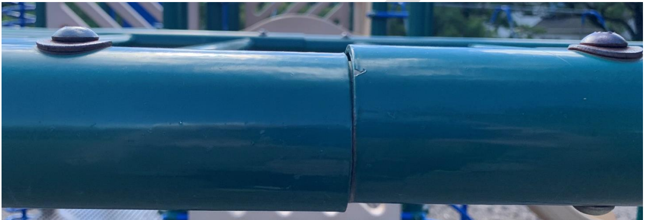
Figure 34: Section of monkey bars with minor misalignment
