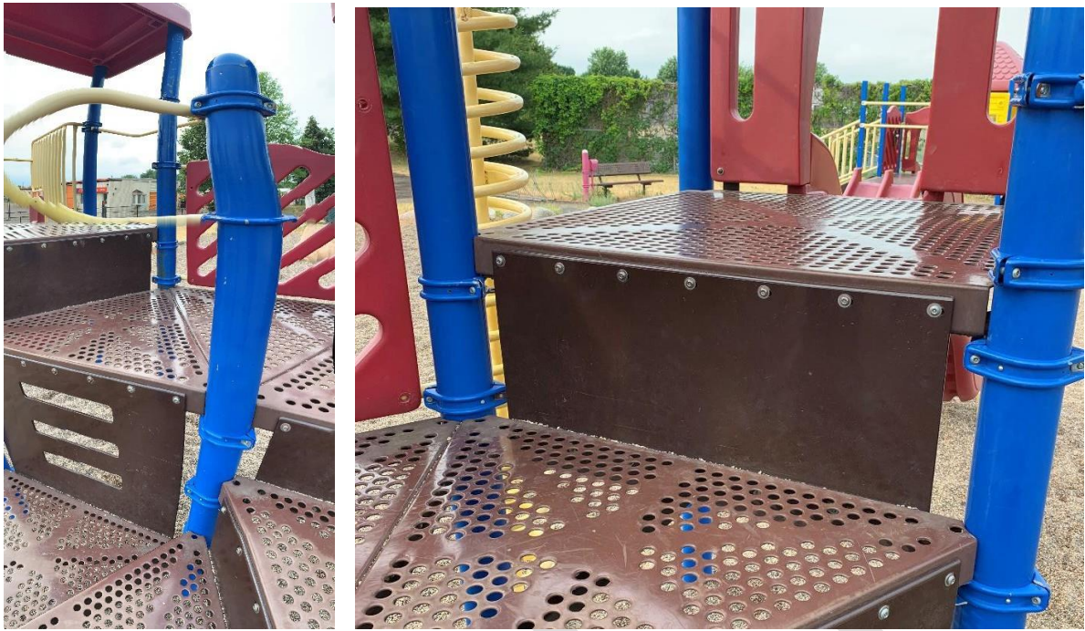
Figures 51-52: Transfer Surfaces on the Larger Playground at Riverdale Park (note that the picture on the left is part of a vertical panorama and is compressed vertically and angularly distorted)
