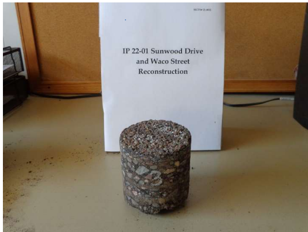
Photo # 3. Core SB-03, 13+00 Sunwood Drive.
