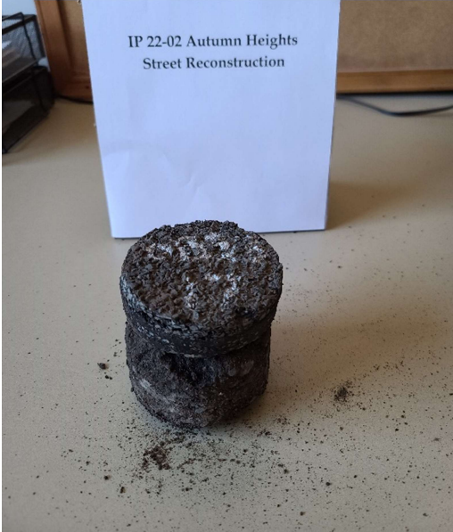
Photo # 17. Core SB-17, 9+00 168 th Lane.
