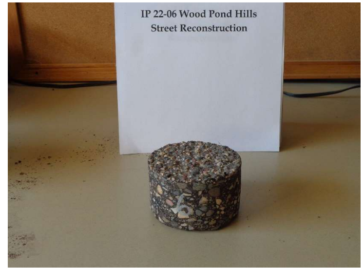
Photo # 6. Core SB-06, 12+00 Junkite Street.
