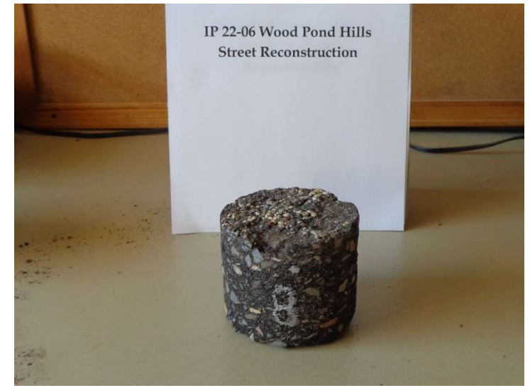
Photo # 8. Core SB-08, 0+50 145 th Court.
