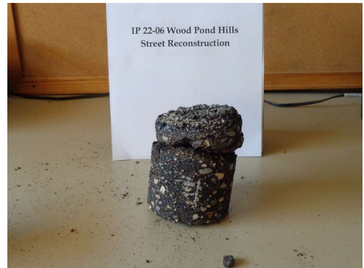
Photo # 4. Core SB-04, 0+50 Junkite Street
