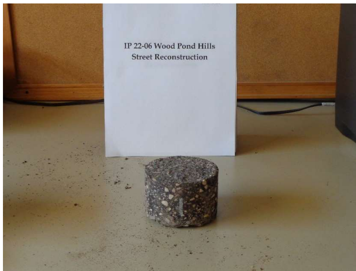
Photo # 1. Core SB-01, 2+50 Krypton Court
