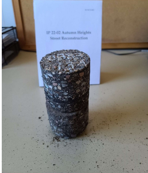
Photo # 13. Core SB-13, 35+50 167 th Lane NW.
