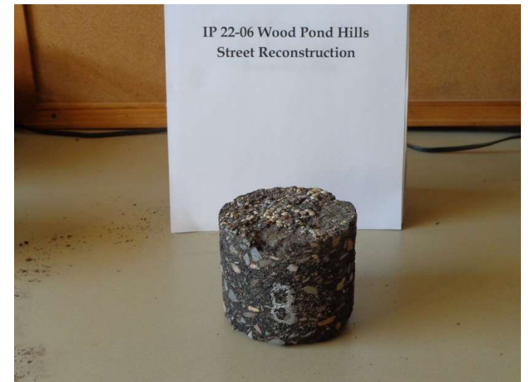
Photo # 8. Core SB-08, 0+50 145 th Court.
