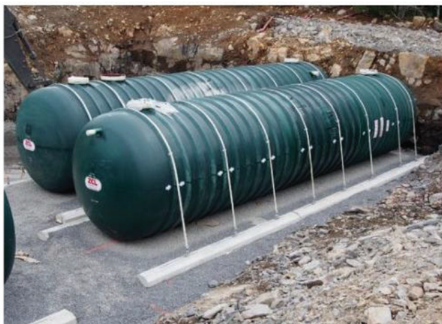
Exhibit 3: Example underground fiberglass storage tanks (Xerxes).
