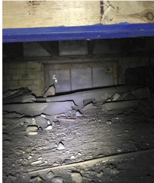
Figure 42 – Exterior Basement Window
