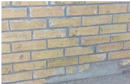
Figure 21 – Mortar Replacement to Fill Voids
