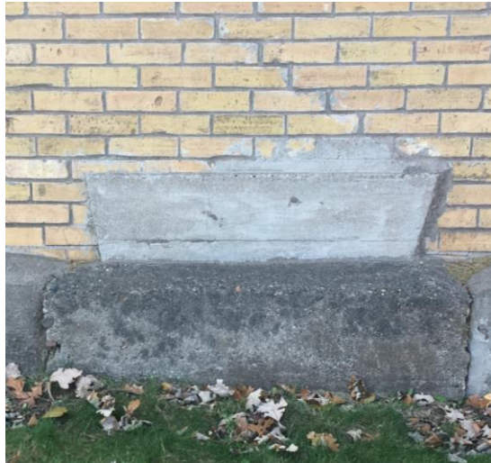
Figure 30 – South Elevation Window
